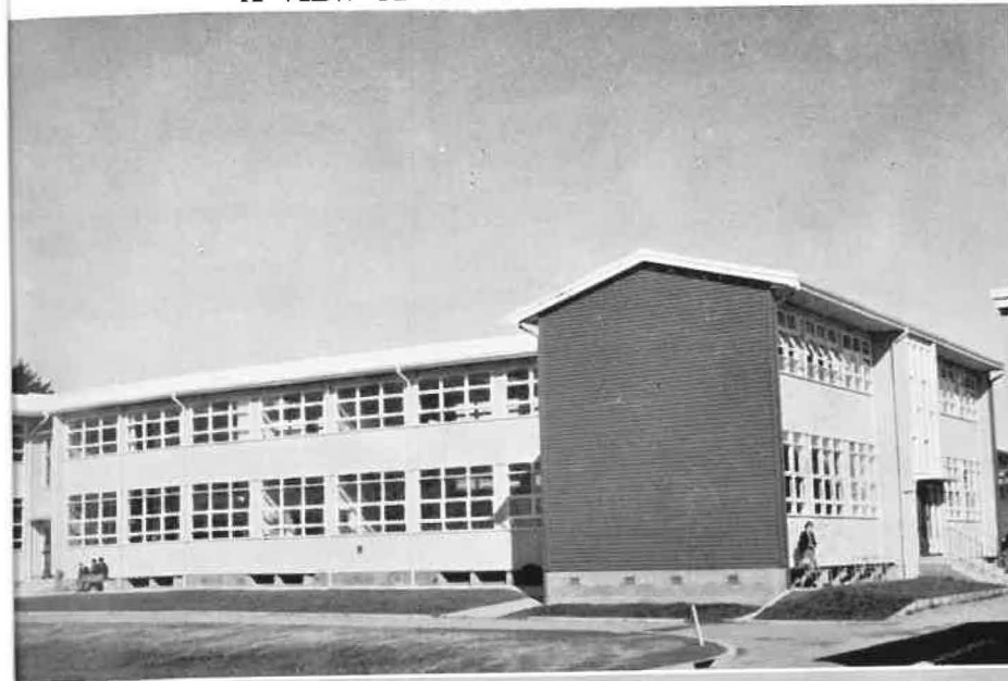
A VIEW OF THE MAIN BLOCK
