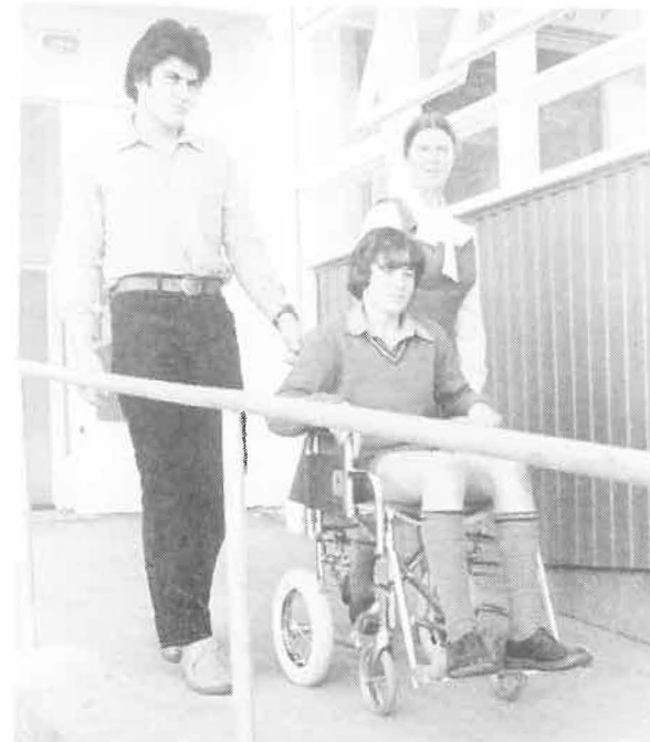
Shane Hurliman (Service Committee), Mrs J. Munro (School Nurse) and Paul Robinson test one of the ramps constructed this year to allow disabled students easy access to ground floor classrooms
