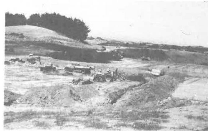
Construction gets under way.
