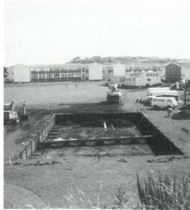
Dig the hole ... but what about that pipe?
