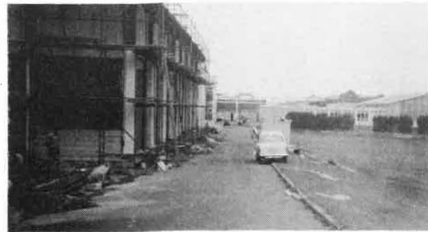
'A' Block construction about 1969 from canteen site.
