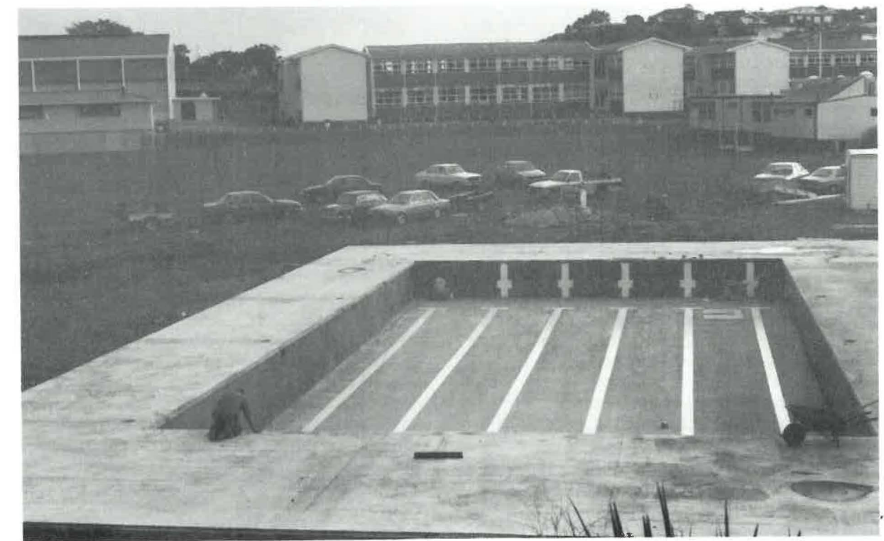
The Swimming Pool under construction.
